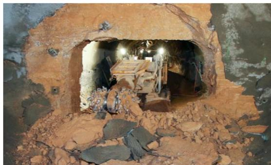
*U1a dual-headed mining breakthrough: Two mining crews working over 960 feet underground finish tunneling toward each other to meet in the middle.*
